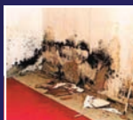
MOLD DAMAGE
